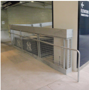
Yankee Stadium - Stairs & Rails
